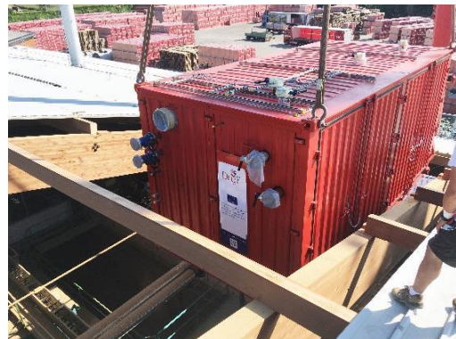
Figure 17: Lifting heat pump container
