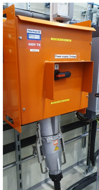
Figure 33: Power supply for the open loop heat pump system (left: for stage one; right: for stage two).
