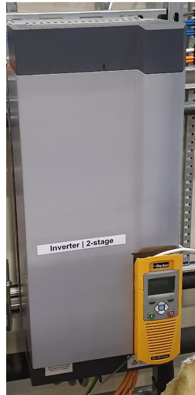
Figure 32: Inverter for power supply to the compressors: stage one with 135 kW (left) and stage two with 75 kW (right)
