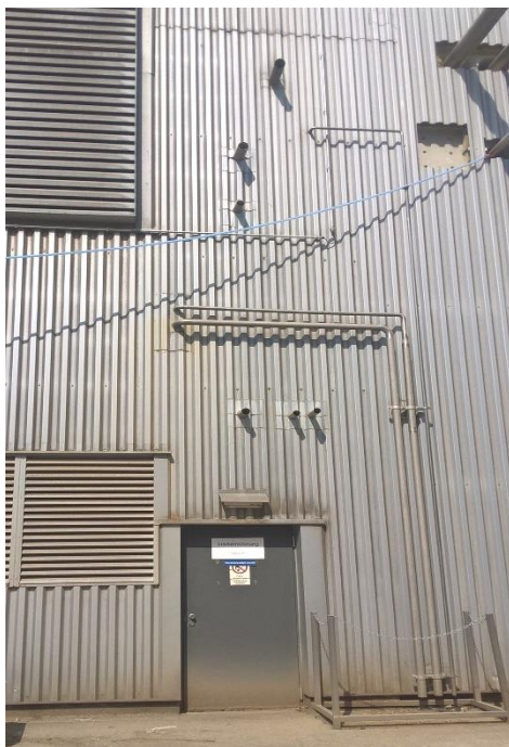
Figure 8: Piping/connections on the outside of the Agrana factory (left: without the heat pump demonstrator, right: including the container of the heat pump demonstrator)
