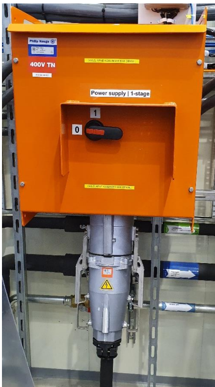
Figure 33: Power supply for the open loop heat pump system (left: for stage one; right: for stage two).
