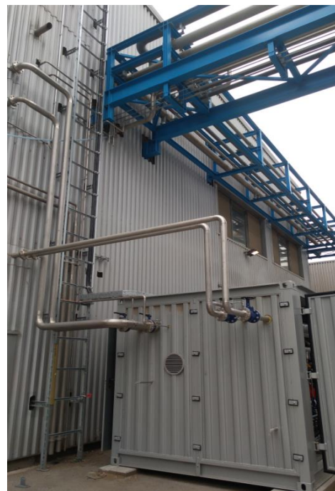
Figure 8: Piping/connections on the outside of the Agrana factory (left: without the heat pump demonstrator, right: including the container of the heat pump demonstrator)
