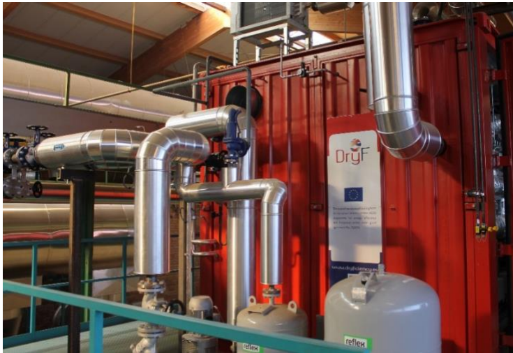
BU: DryFiciency high-temperature heat pumps were commissioned in three applications and tested in an industrial environment. System at Wienerberger AG in Uttendorf © AIT / Schneeberger
